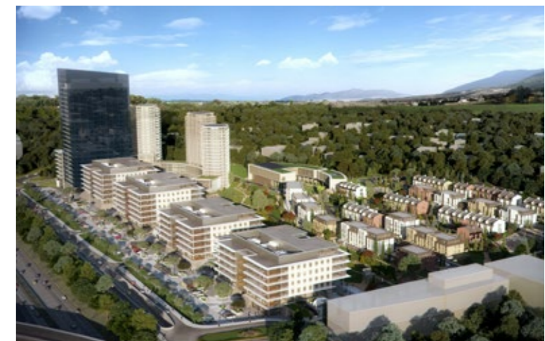
Garitage Park, developer: Garitage Investment Management
