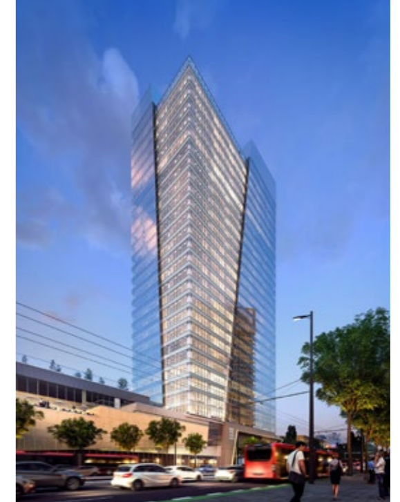
Nivy Tower, developer: HB Reavis
